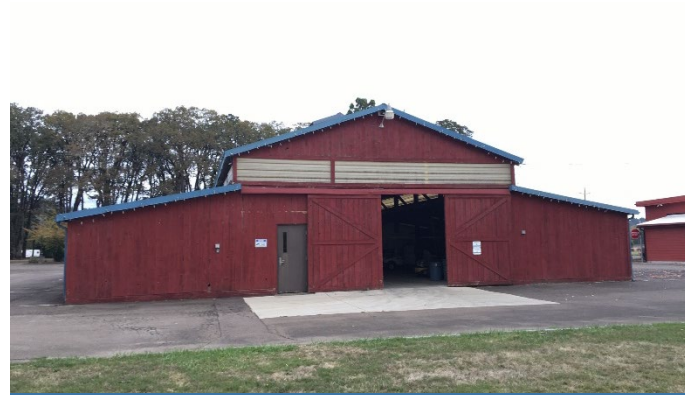
Benton Barn Upgrades
