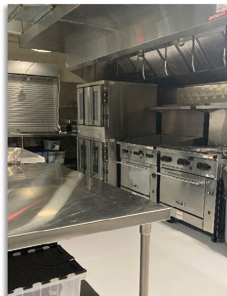
Benton County Fairgrounds Commercial Kitchen
