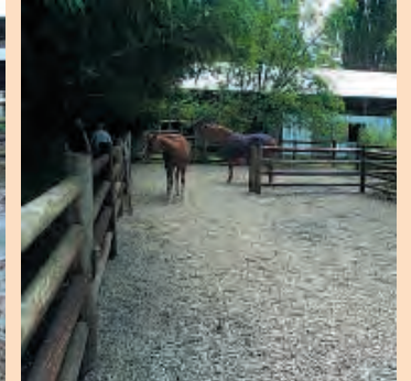
Corral and happy horses after installation of gravel. (Photo courtesy of Kitsap Conservation District)
