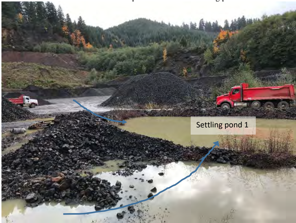
From settling pond 1, water is conveyed easterly via culvert under access road to bioswale. From bioswale, water is conveyed back westerly under the access road and discharges into a vegetated buffer
