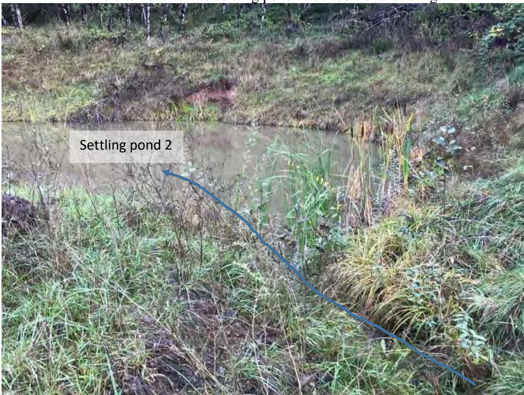
The ditch drains into settling pond 2 for additional settling.
