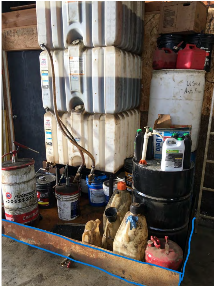
Secondary containment for all oil in the shop, blue line represents an oil catch.
