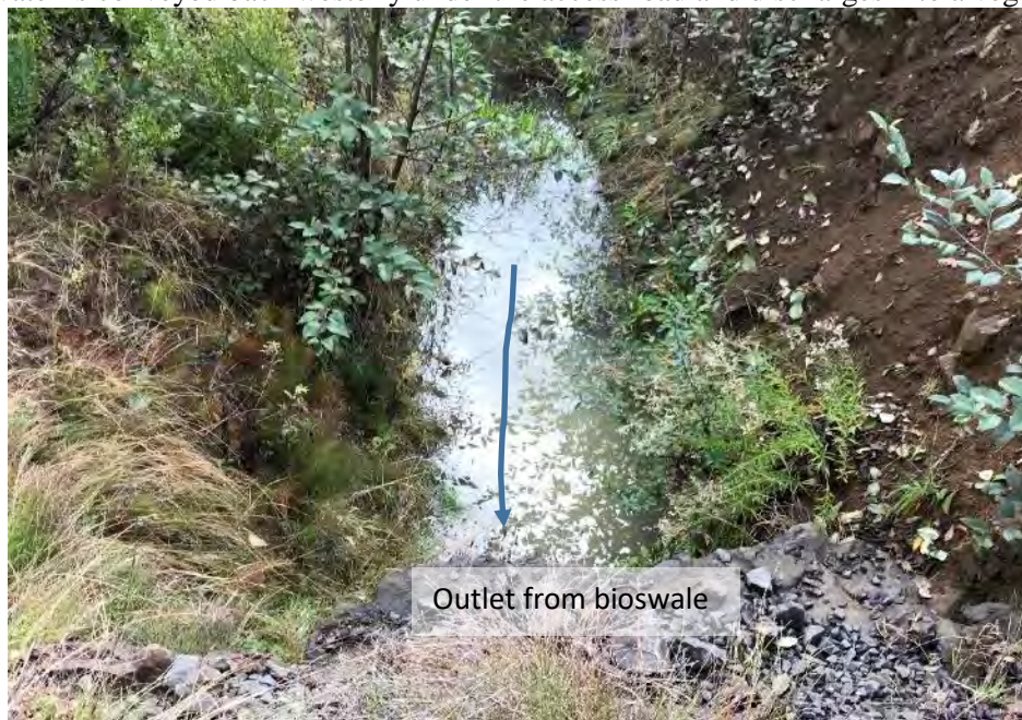
From settling pond 1, water is conveyed easterly via culvert under access road to bioswale. From bioswale, water is conveyed back westerly under the access road and discharges into a vegetated buffer
